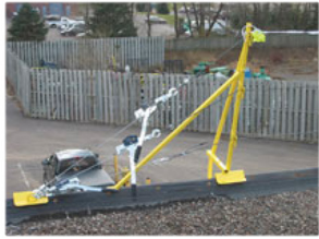
Simple ratchet pullers tension cable around the entire system.
