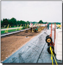
Stanchion rigged for flat commercial job.
