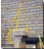
Stanchion rigged for parapet wall.
